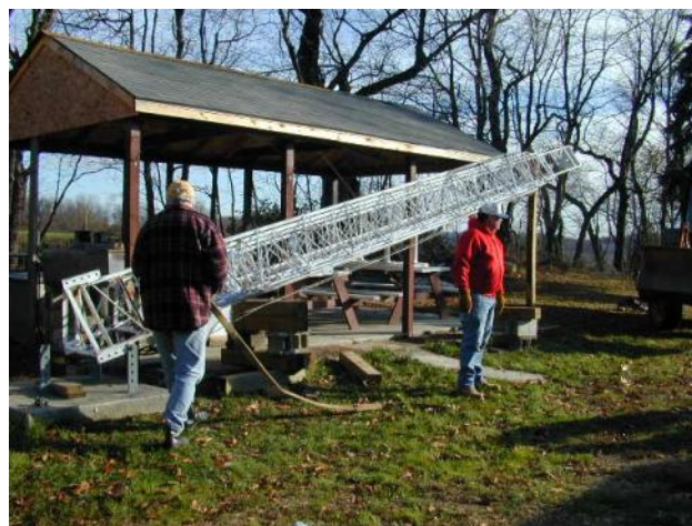
Getting it up without a crane took some doing
